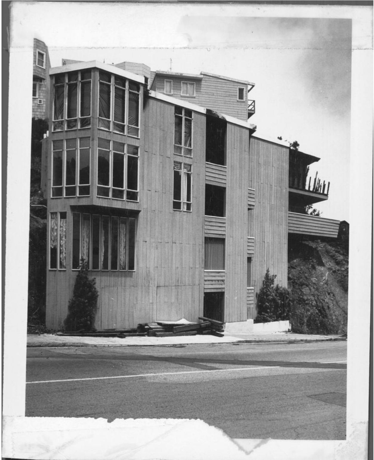
310 Corbett, June 1967, after a fire, before purchase and repair by Chamberlain Note: Shingles not part of the original design.
